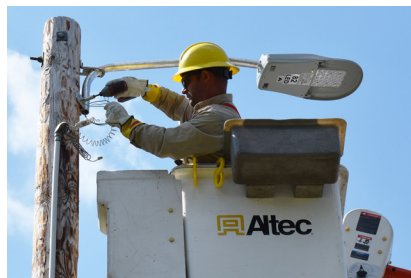
CWEC Service Foreman John Bestul installs a new LED light fixture as part of the Stockbridge-Munsee light project.
