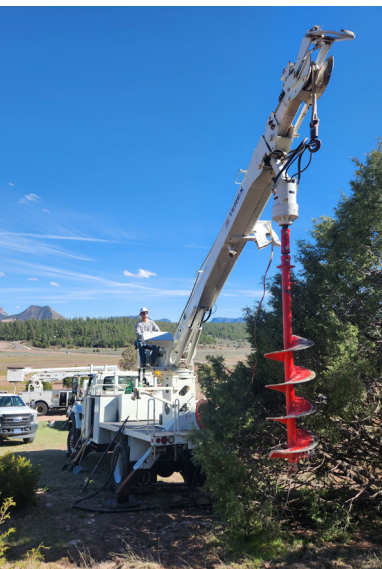
Left to right: Jarret Brow operates a digger to dig a hole for a new power pole; Alex Lutz (seated on the truck) helps install a line of new power poles on the Navajo Nation; Jarret Brow does work at the top of a newly installed power pole that will be used to bring electricity to residents of the Navajo Nation; A line of newly installed power poles on the Navajo Nation that will bring electricity to the residents of the Navajo Nation. The work to install the poles was part of the Light Up Navajo IV Project.
