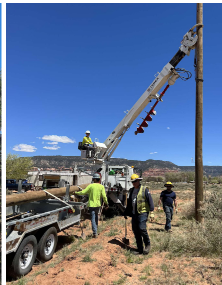
Left to right: Jarret Brow operates a digger to dig a hole for a new power pole; Alex Lutz (seated on the truck) helps install a line of new power poles on the Navajo Nation; Jarret Brow does work at the top of a newly installed power pole that will be used to bring electricity to residents of the Navajo Nation; A line of newly installed power poles on the Navajo Nation that will bring electricity to the residents of the Navajo Nation. The work to install the poles was part of the Light Up Navajo IV Project.
